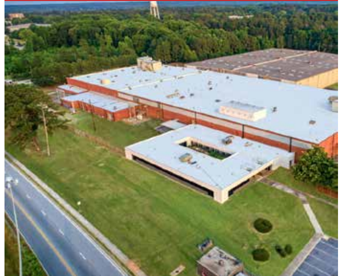
Ascend Elements battery recycling facility in Covington, GA
