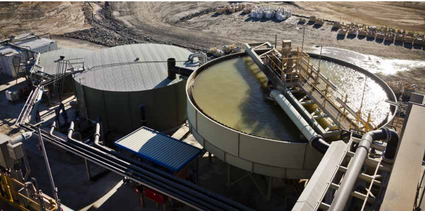
Processing plant at a lithium mine in Western Australia
