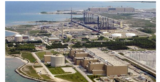
Bruce Power site – home to the existing Bruce Nuclear Generating Station
