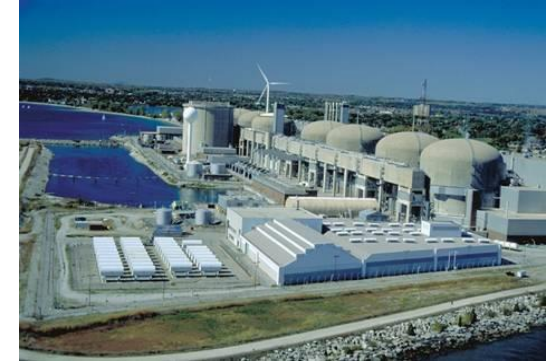
Pickering Nuclear Generating Station
