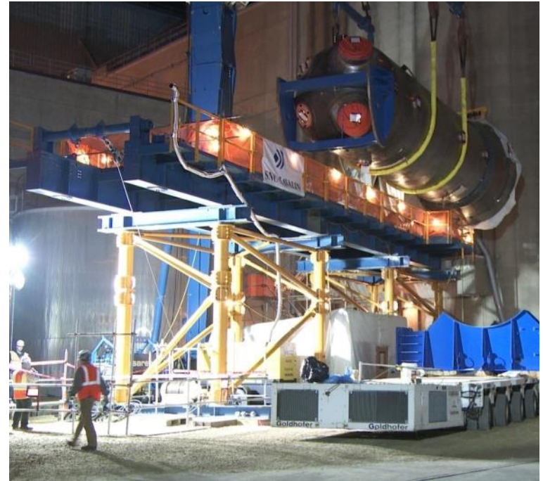
Steam generator replacement in progress
