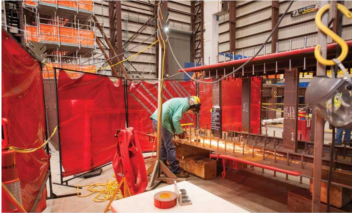
Welding and Rewelding at Vogtle
