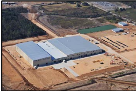
Structural Modules from CBI - Lake Charles, LA
